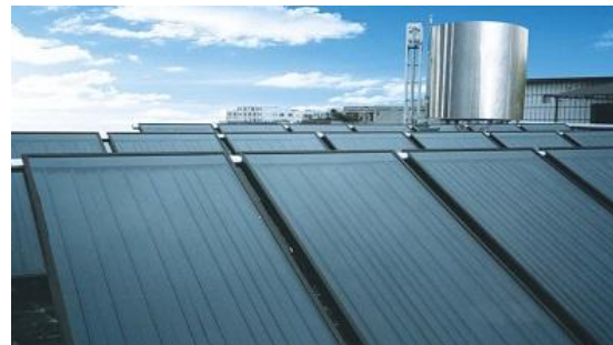
Figure 1. Flat-plate collectors
