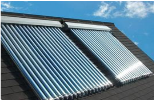
Figure2. Evacuated tube collectors
